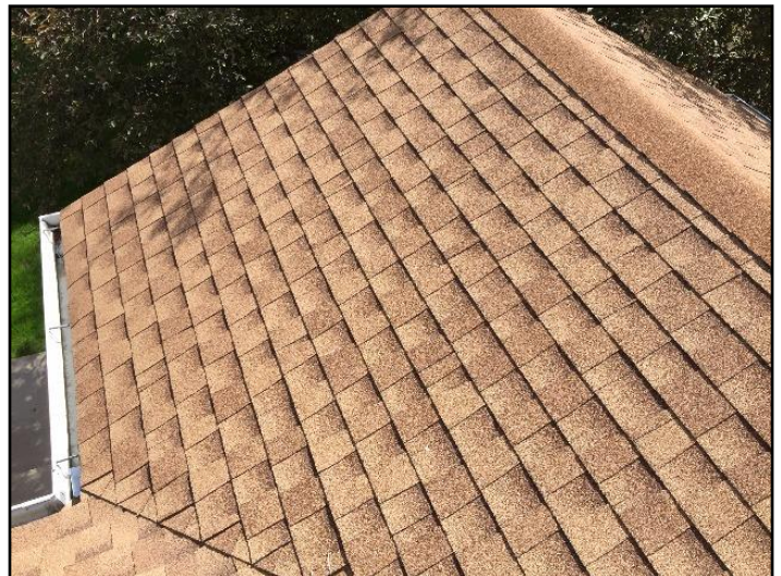
4. Asphalt shingles
